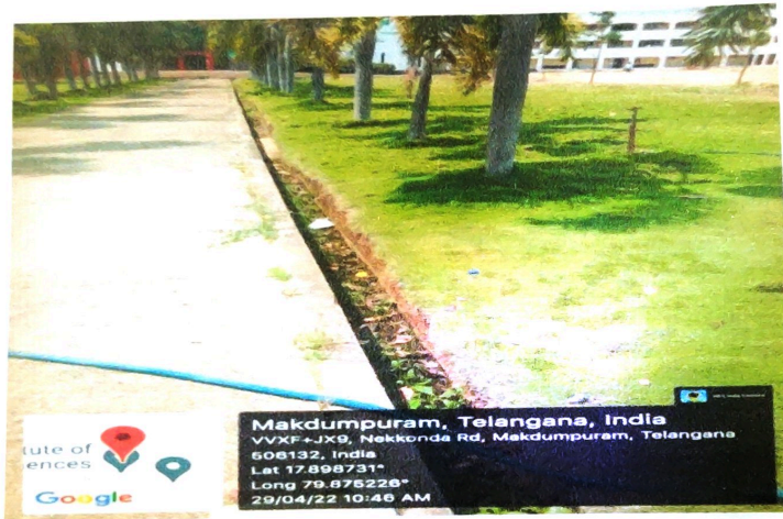
Surface drains collecting liquid waste in the campus
